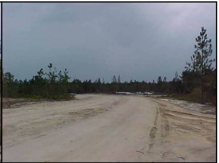
Looking towards Lee Road along Longreen Parkway
