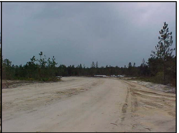
Looking towards Lee Road along Longreen Parkway
